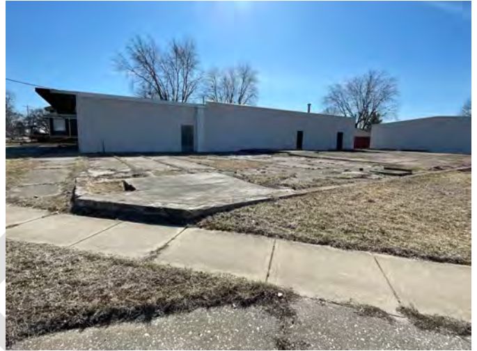
Deteriorating slab foundation adjacent to the vacant commercial storefront at 1702 Grand Avenue.
