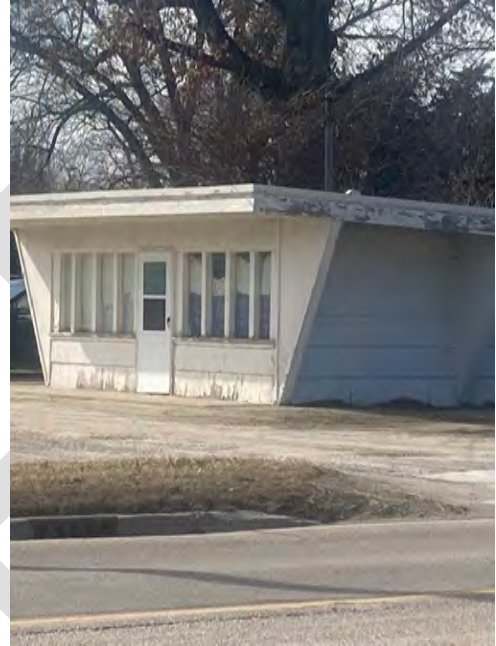
Deteriorated commercial structure at 2138 Grand Avenue. (Worn siding, window framing, and fascia.)
