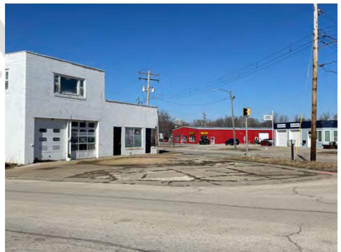
Deteriorated, vacant commercial building (damaged roll up doors, windows, and tuckpointing) and site improvements (cracked and crumbling parking lot pavement) at 1690 Grand Avenue.
